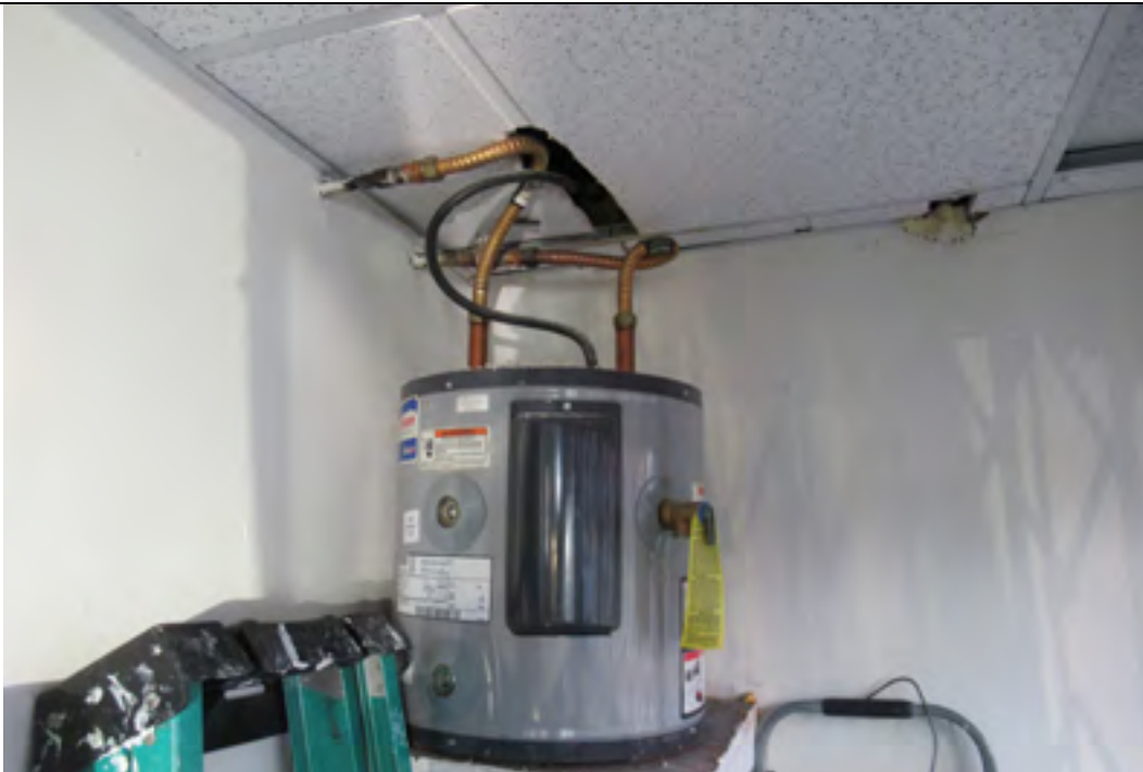
View of the 6-gallon water heater supplying 1914 West 8 th Street.
