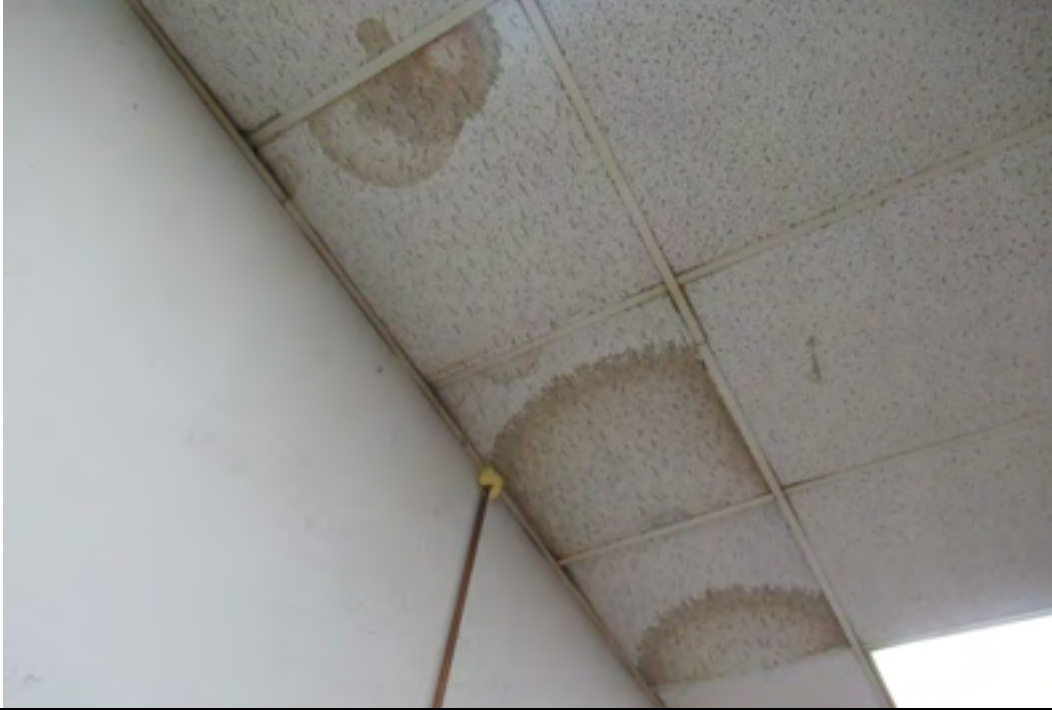
View of limited areas of previous moisture damage observed on the acoustic ceiling tiles at 1914 West 8 th Street.
